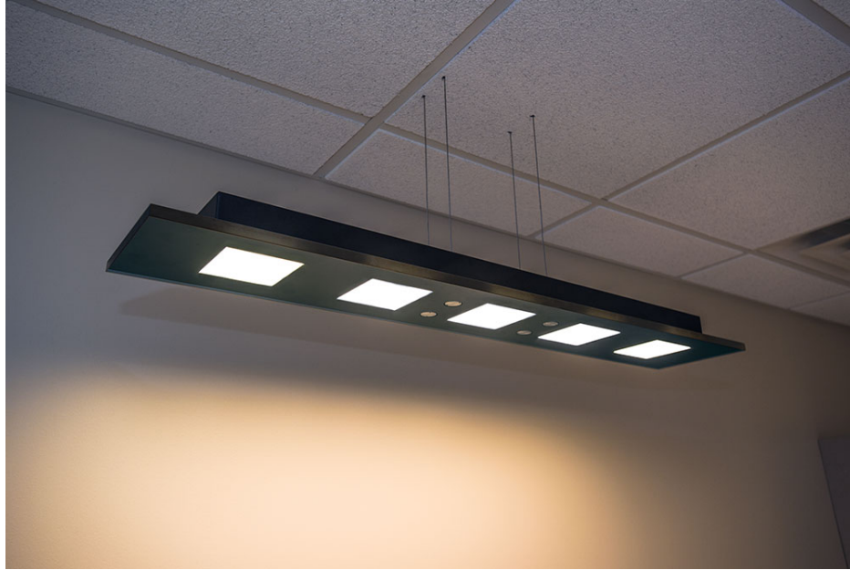
Figure 13. Closeup of the Designplan "Blade" luminaires suspended in the copy room. Photo courtesy OLEDWorks LLC and DeJoy Knauf & Blood, LLP.
