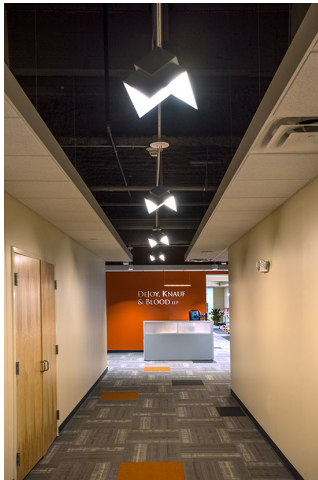
Figure 16. Entry corridor to DKB offices showing four Visa Lighting Petal™ pendants and a five-panel OMLED One s5 pendant above the reception desk. Photo courtesy OLEDWorks LLC and DeJoy Knauf & Blood, LLP.
