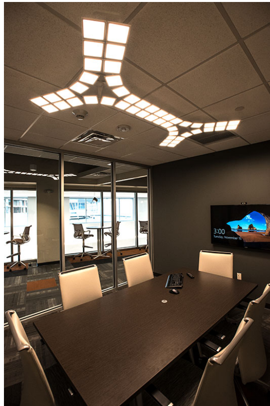
Figure 9. Smaller conference room showing 48-panel Acuity Brands Winona® Trilia™ pendant. Photo courtesy OLEDWorks LLC and DeJoy Knauf & Blood, LLP.
