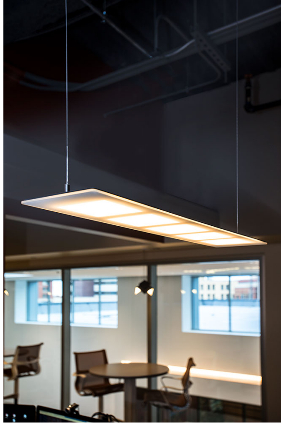
Figure 17. Closeup view of the OMLED One s5 pendant suspended above reception desk. Photo courtesy OLEDWorks LLC and DeJoy Knauf & Blood, LLP.
