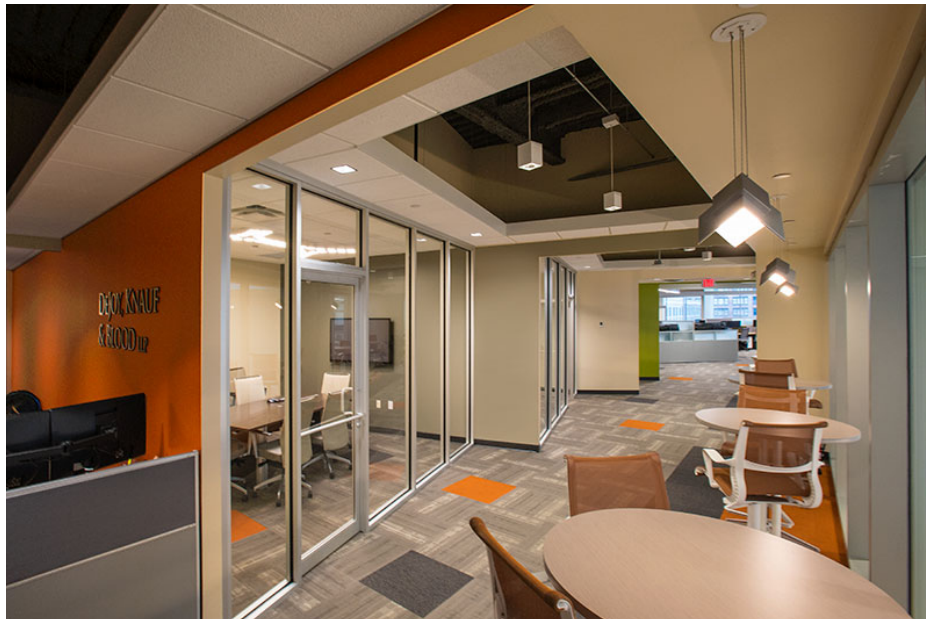
Figure 15. Visa Lighting Petal™ OLED pendants suspended above high-top tables in a casual lounge area off a main corridor. A small conference room equipped with OLED configuration is visible through the windows on the left. The square recessed downlights and cube pendants use LED sources. Photo courtesy OLEDWorks LLC and DeJoy Knauf & Blood, LLP.
