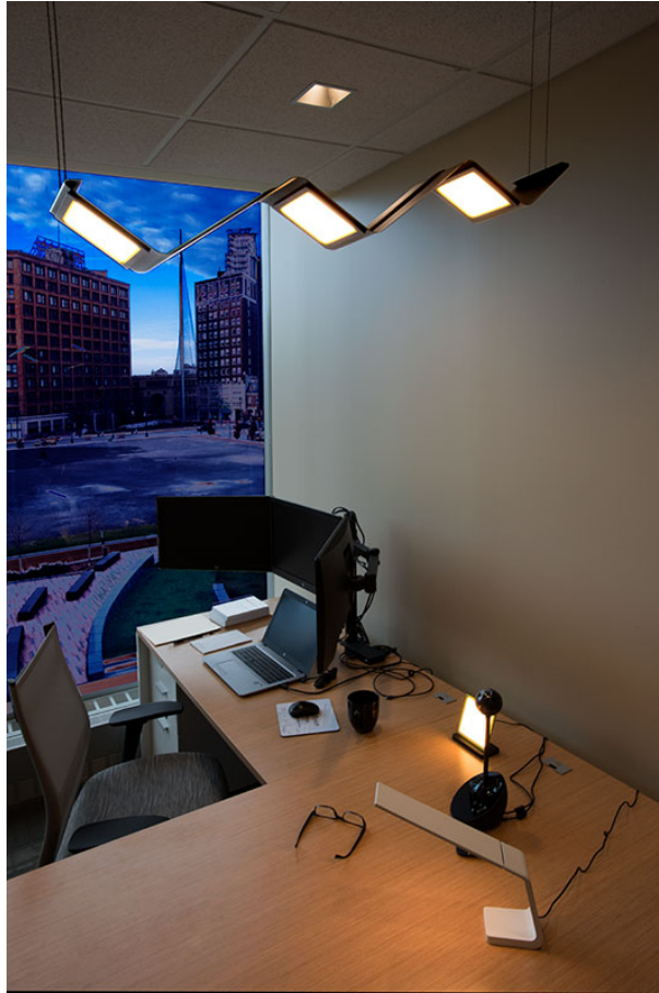
Figure 4. Perimeter office, showing recessed LED downlights, the Visa Limit™ OLED pendant light, and OLED Devices task light (in foreground). The glowing square on the desk is an award with printed text and images backlit by a single OLED lighting panel. Photo courtesy OLEDWorks LLC and DeJoy Knauf & Blood, LLP.
