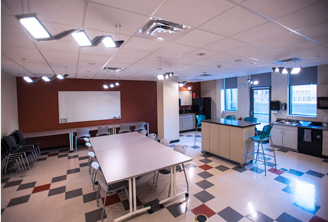
Figure 10. The TeamDKB break room showing the recessed square LED downlights and the playful Visa Limit™ pendants. Photo courtesy OLEDWorks LLC and DeJoy Knauf & Blood, LLP.
